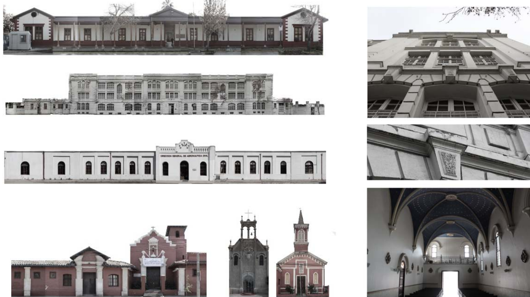
Figures 13 – 21: Some cases of non-safeguarded architectural heritage at Estación Central Commune: Ancient Agriculture Practical School, School República de Venezuela, Aeronautical Technical School, Amengual Convent, Santiago Apóstol Chapel, and Las Carmelitas' Chapel. Nowadays this architecture is in use, but still vulnerable of demolition. Photographs taken by Dicyt Research Project Team
